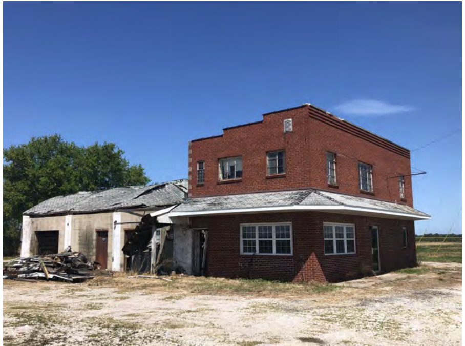
The building as it appeared in August 2021. Southeast corner.
