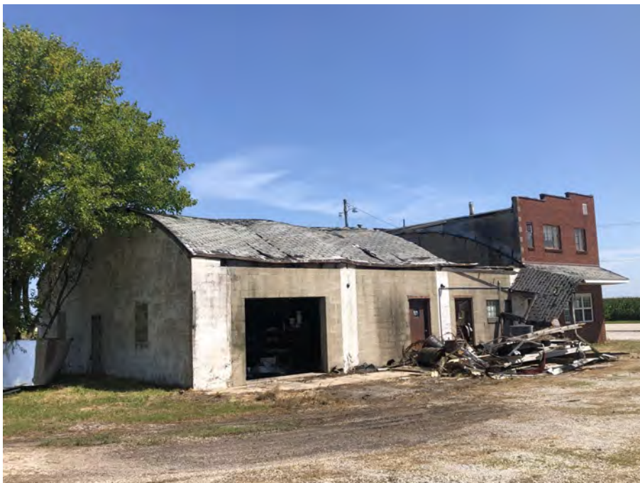
The building as it appeared in August 2021. Southwest corner.
