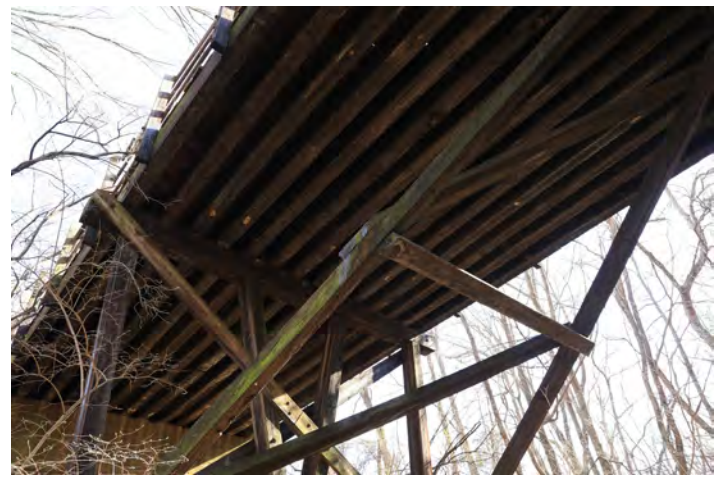
Diagonal bracing between the first and second bents
