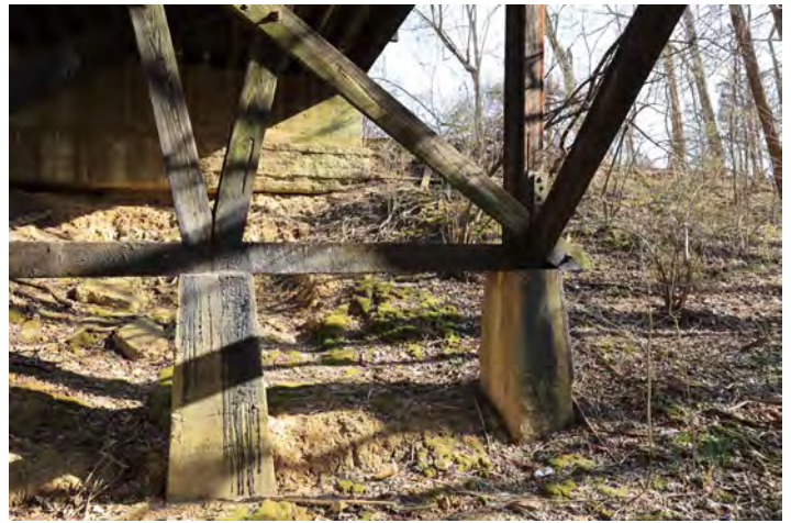
Closeup of the footings supporting the bents
