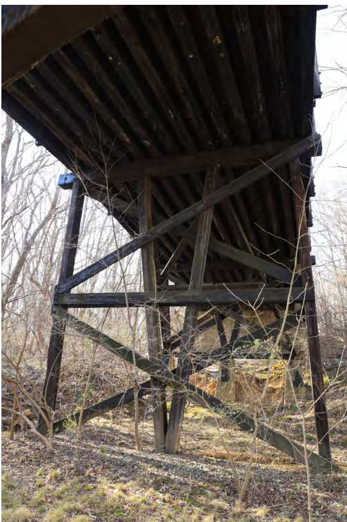
The bents meet the stringers underneath
