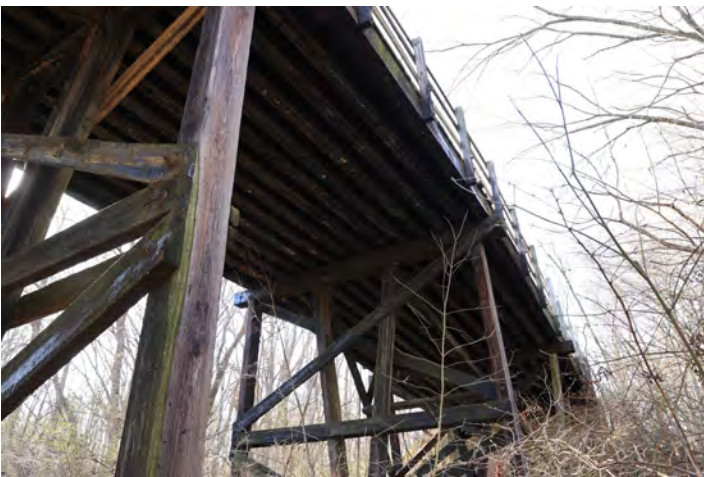
The bents meet the stringers underneath
