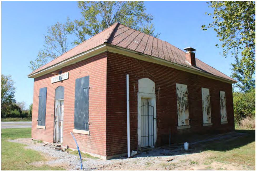
Southeast corner. The side door was added at a later date. Note the vent and cleanout pipe for the restroom added in 1988.
