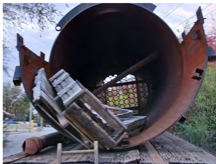
View of boiler from fire box end, looking forward, PRR T1, No. 5550, 4-4-4-4
