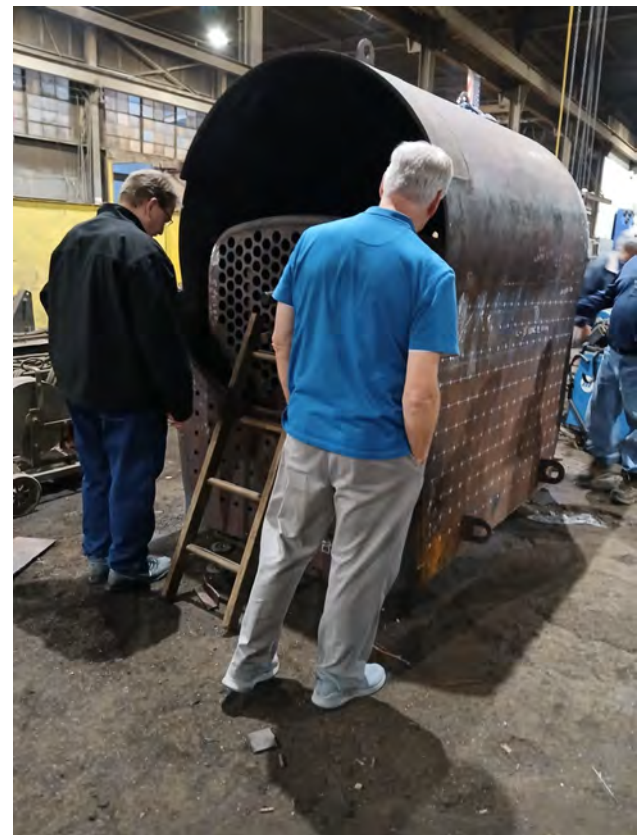
Inspecting fire box for replacement F&J #112 boiler,
