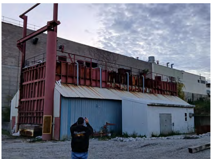
Gas fired heat treatment oven
