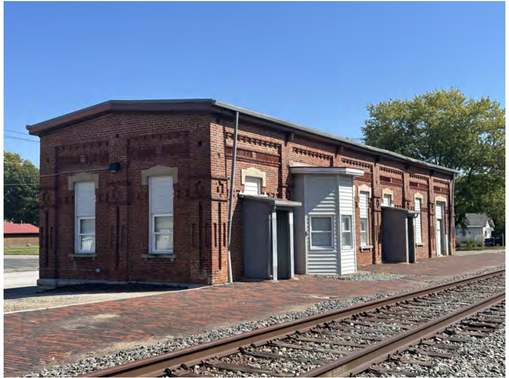
View of the Salem, Illinois B&O/Chessie/CSX depot as it appeared in September 2025. Photo by Jeff Cooper
